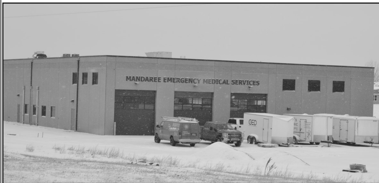
Pictured above is our new Mandaree Emergency Medical Service Building.
