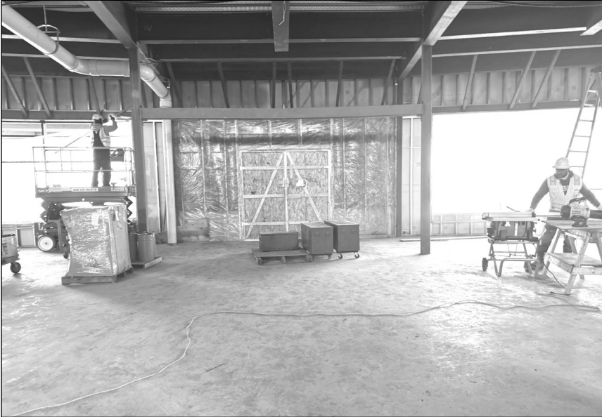
The main entrance will be here.
