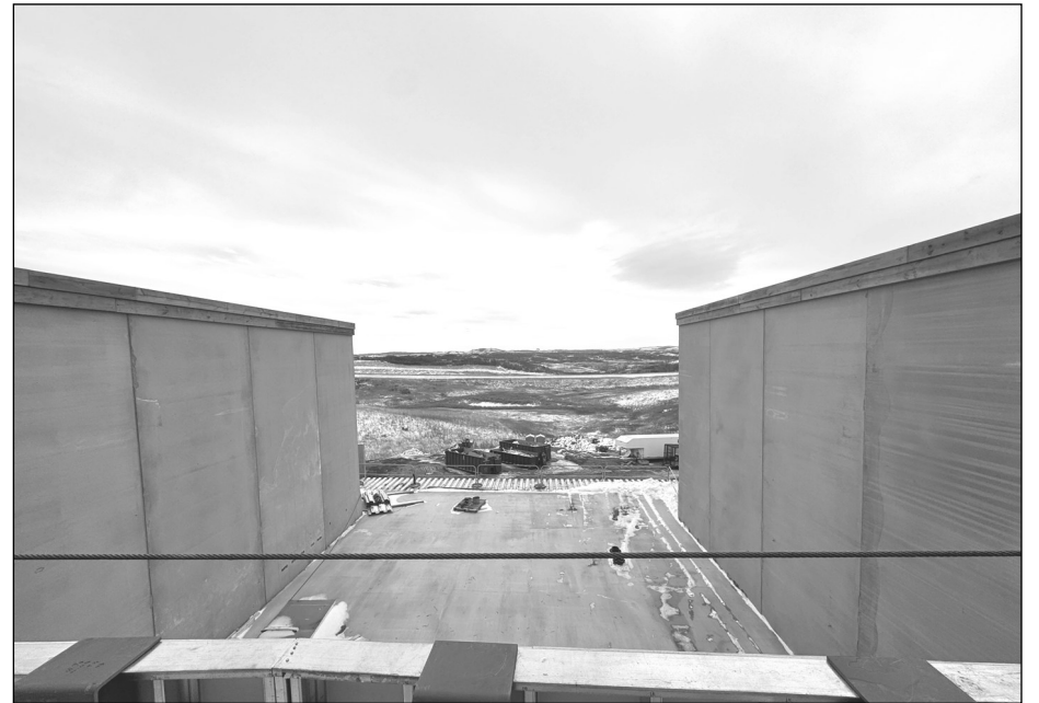
Observation deck facing south towards Eagles Nest. The walls inside will be the memorial hall.
