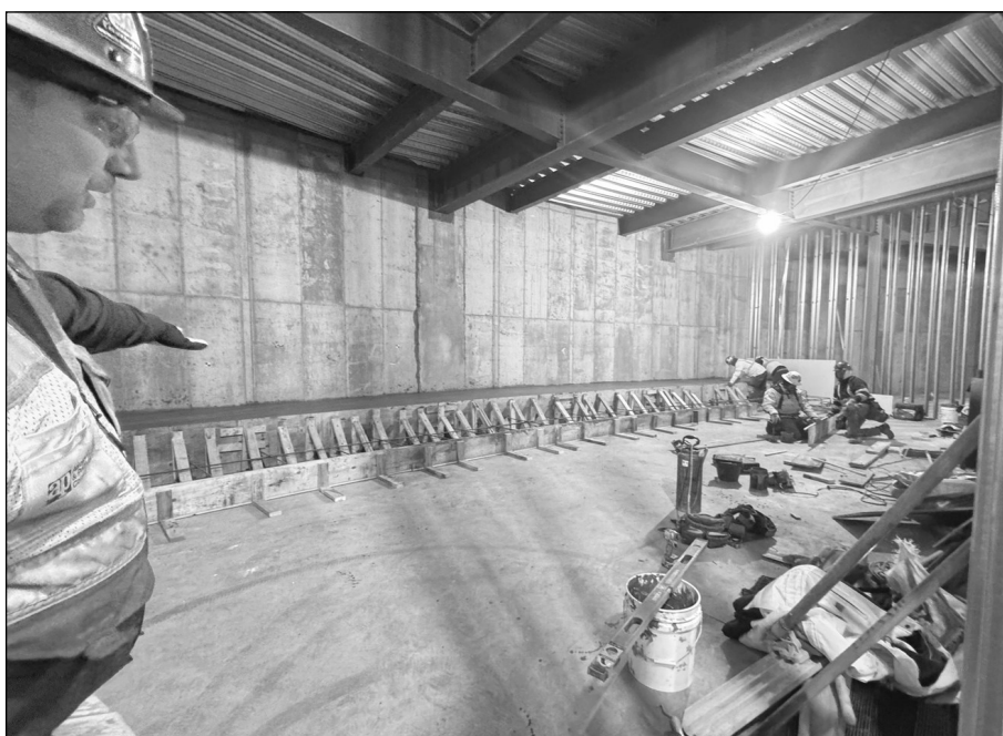
Lecture hall will be here in this area.
