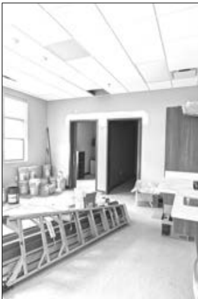
Physical therapy room still under construction.
