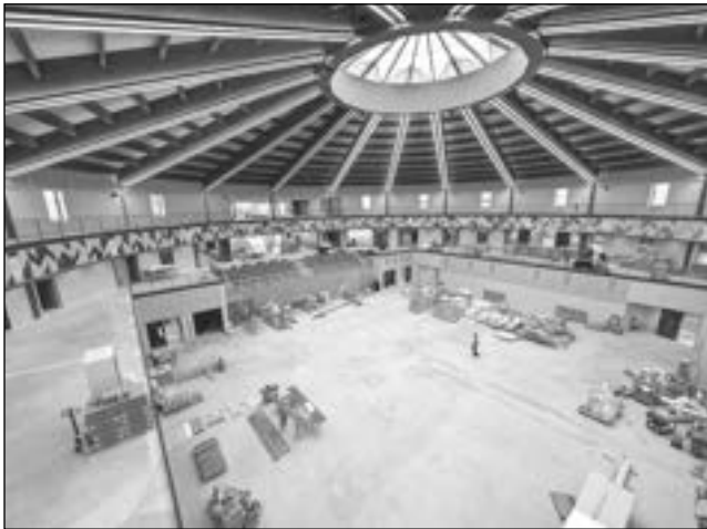
Here is a view of the hall from the top.
